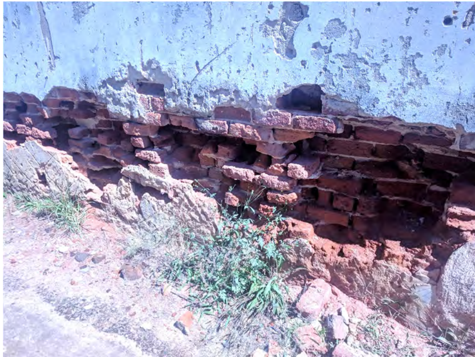
Photo #5 – Building 405 - Missing and Damaged Brick in Southwest Exterior Wall
