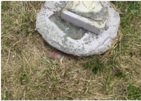
Old well needs to cap off and secure properly
