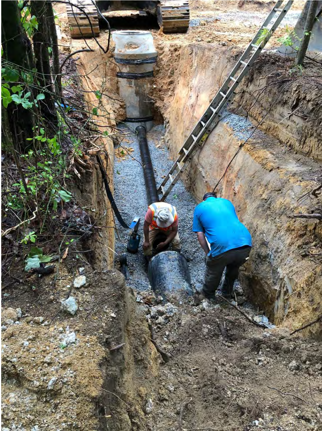
Jack and bore behind the pond being installed.
