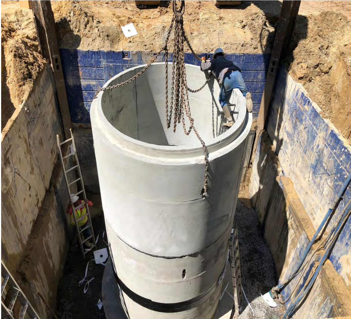
The wet well for the pump station being installed.
