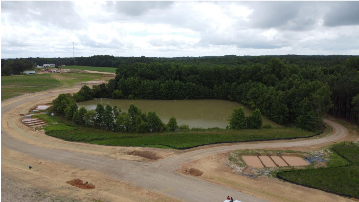
Industrial Park Drive and the road to the pump station.
