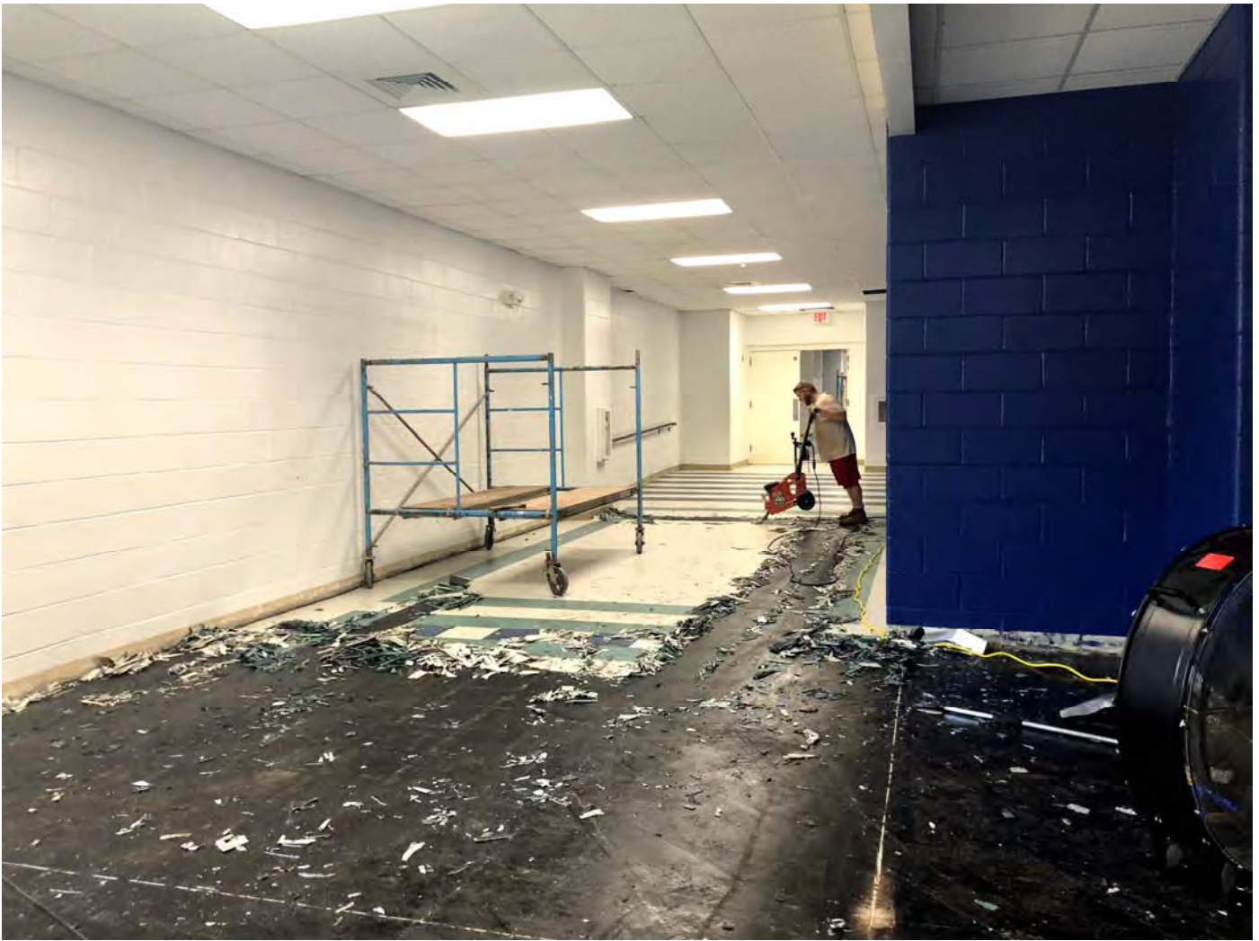
Existing hall to main building: Flooring currently being removed.
