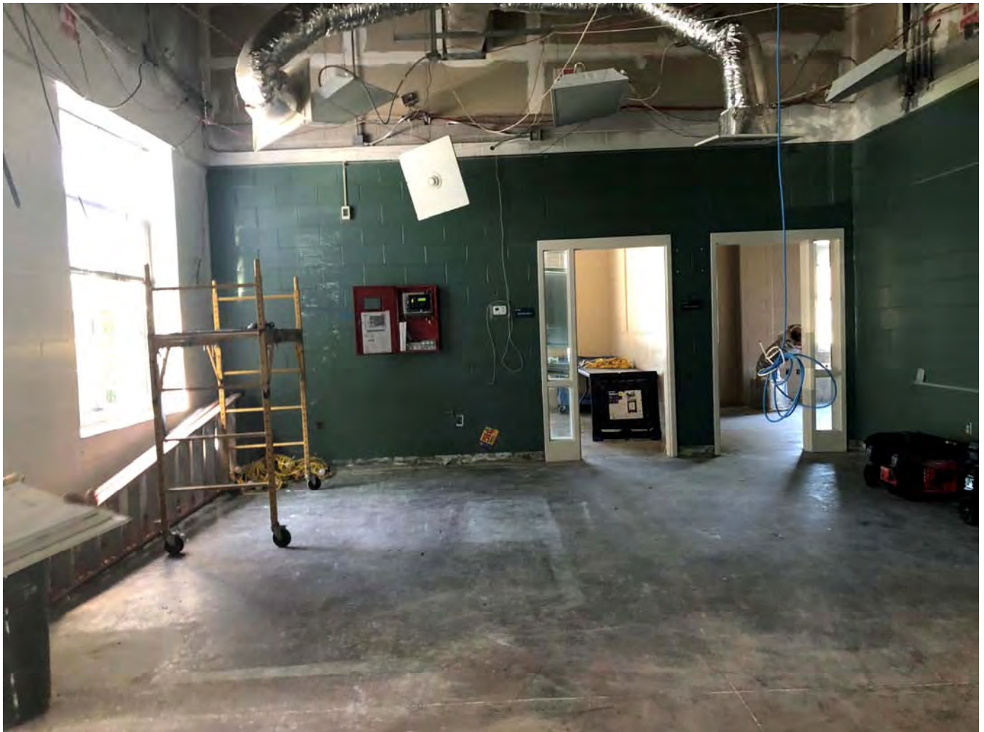
Existing Entry Lobby: Casework, some wall mounted fixtures, ceiling grid and tiles, and VCT flooring have been removed.
