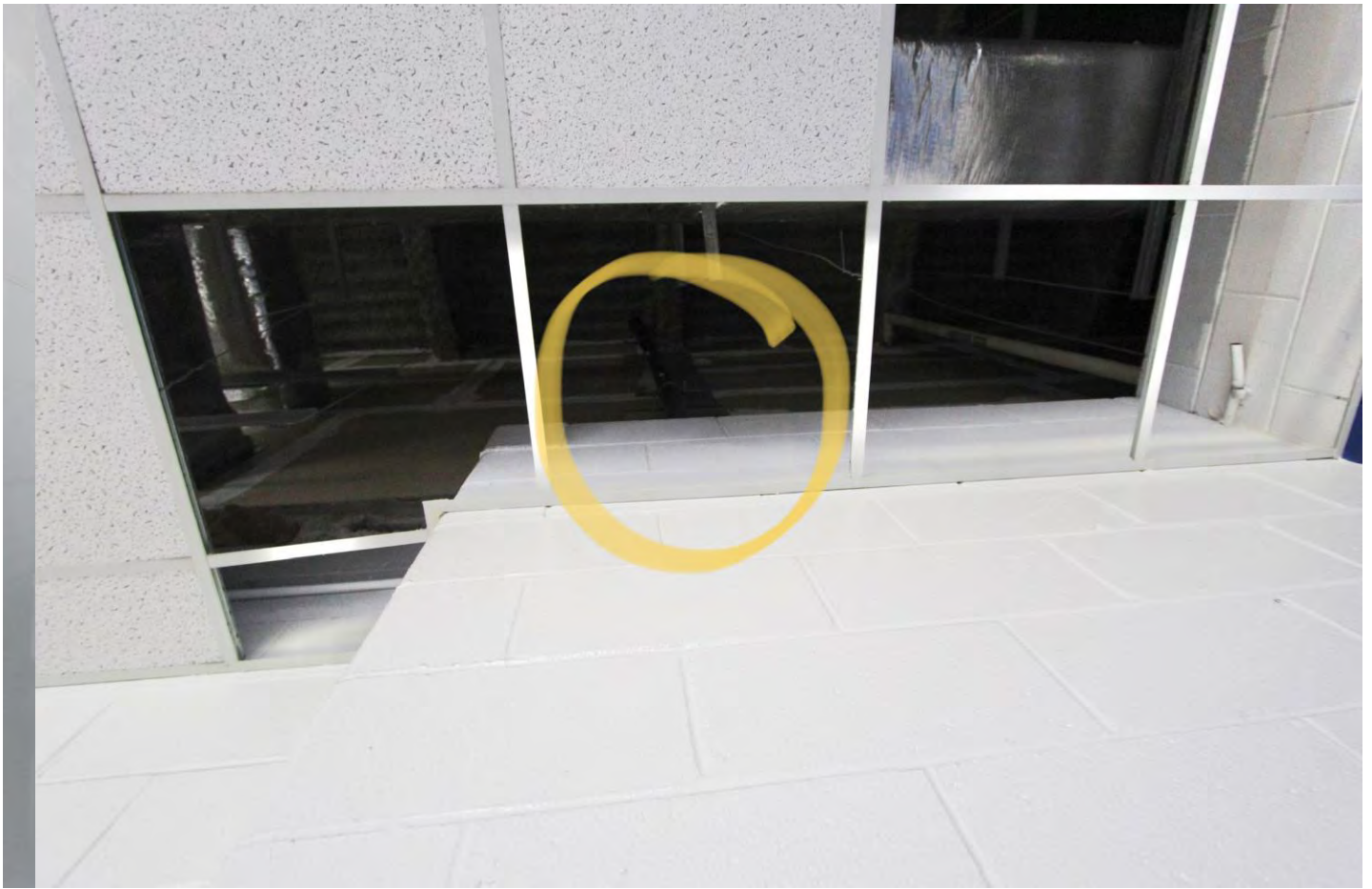
Classroom A120 bumpout is block not gyp, to be demoed and case around pipe
