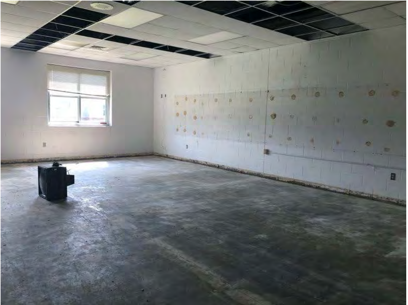
Existing Classroom Demo: Casework, flooring, base, wall mounted accessories, and ceiling tiles have been removed.
